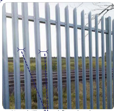
Site drilled and fitted pales are much more susceptible to incorrect pale spacings
