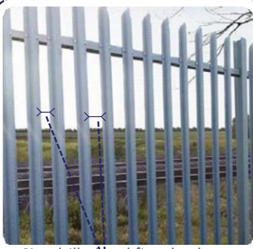
Site drilled and fitted pales are much more susceptible to incorrect pale spacings
